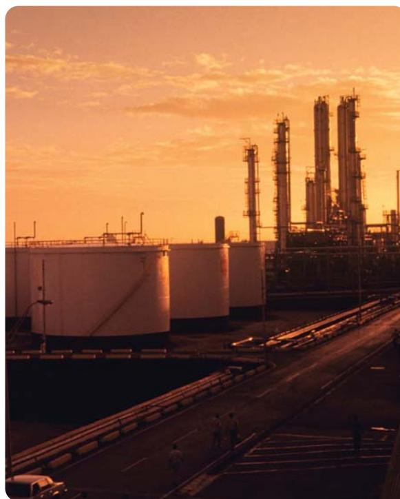
The crude oil in the refinery's storage tanks will be transferred to a blending manifold where it will be blended to the desired composition ratio range predetermined by production. Storage space, or lack thereof is another important problem in many refineries. The more oil that's found, the more tanks become necessary and the more offshoots of the pipeline are needed.
